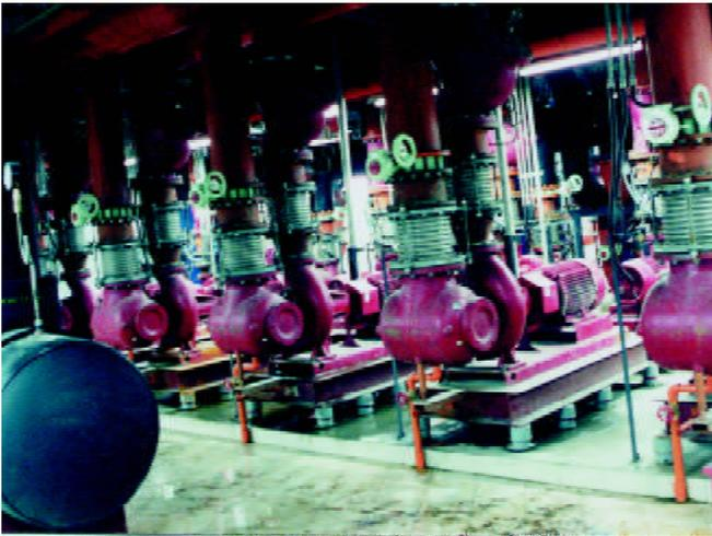
Figure 3: Variable speed pumps are controlled by variable frequency drive control panels.
