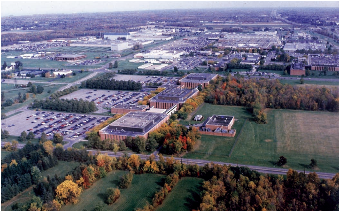
Photo 1: Xerox was able to increase efficiency and interoperability, as well as reduce costs, at its Webster, N.Y., campus by implementing a BACnet-based system. The campus includes research, engineering and manufacturing areas, cafeterias, offices, and conference rooms.
