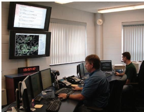
*Sixteen computers and 12 display screens provide the operators of Cornell’s EMCS Operations Center flexible access to all campus systems.*
