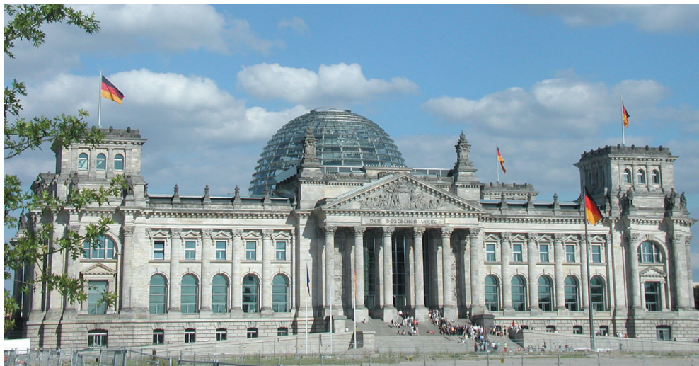
BACnet was installed during a recent renovation of the Reichstag in Berlin.
