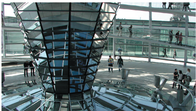
At the Reichstag, many proprietary protocols were tied together via a BACnet/IP-Ethernet network.
