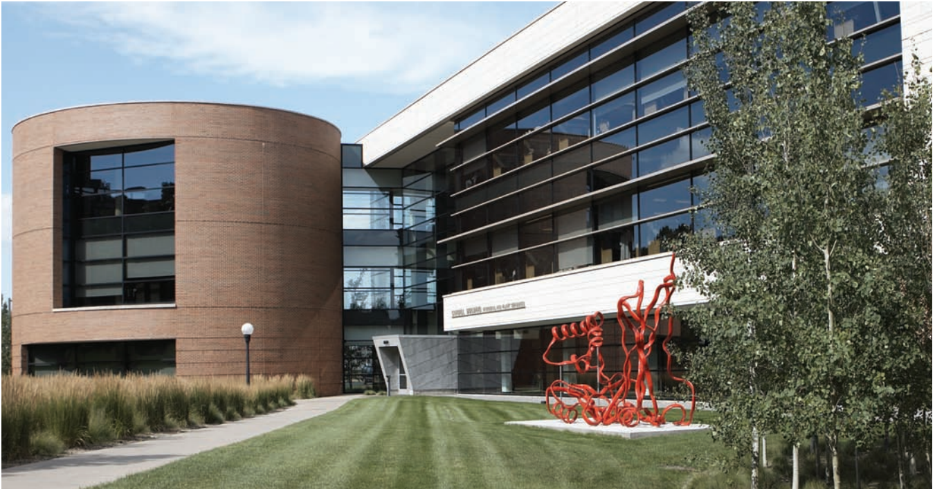
BACnet is used at the University of Minnesota to centralize control over building systems.
