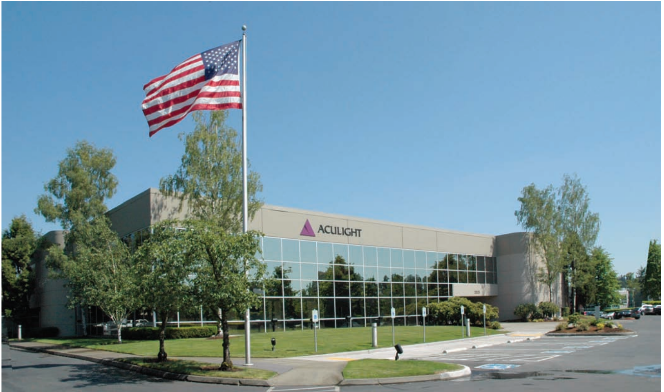
Aculight, a laser manufacturer in Washington, is using BACnet to provide precise temperature and humidity controls to its cleanrooms.
