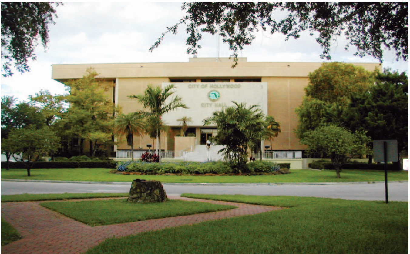
An open protocol controls system enables the City of Hollywood, Fla., to efficiently consolidate and control multiple sites.
