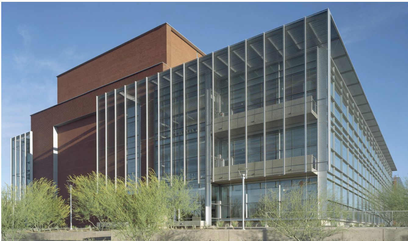
Arizona State University's Biodesign Institute uses BACnet to help optimize building systems.
