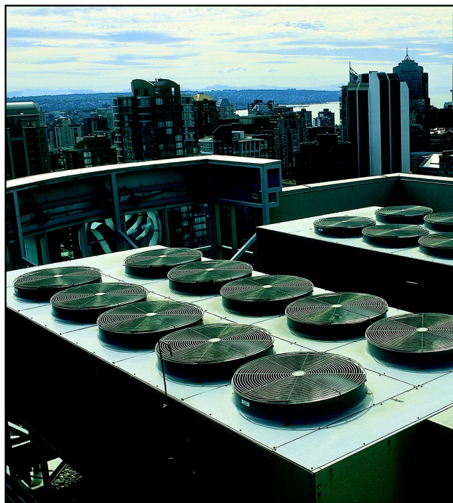
Air-cooled chillers on roof provide cooling for guest rooms.
